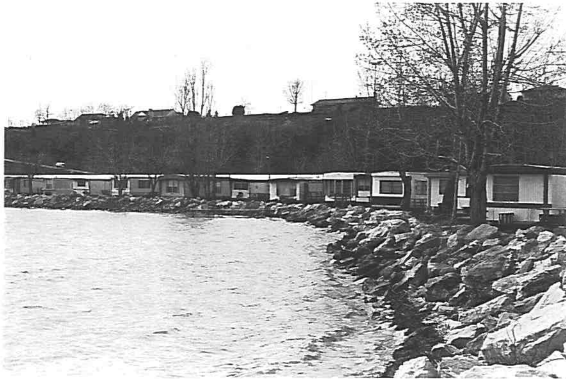
Photo 4 North Shore site, trailers at Booths' Marina
